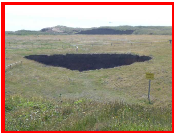
Enlarged sink hole at the former Old Harbour Quarry – detailed view (/0501C01)
