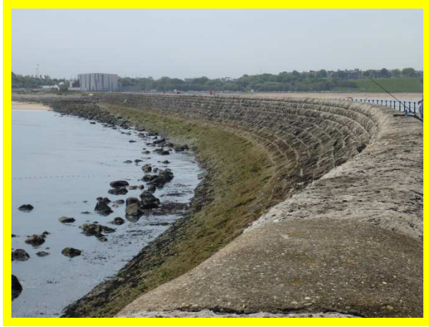
South Pier in overall fair condition along southern face (/0103C01)
