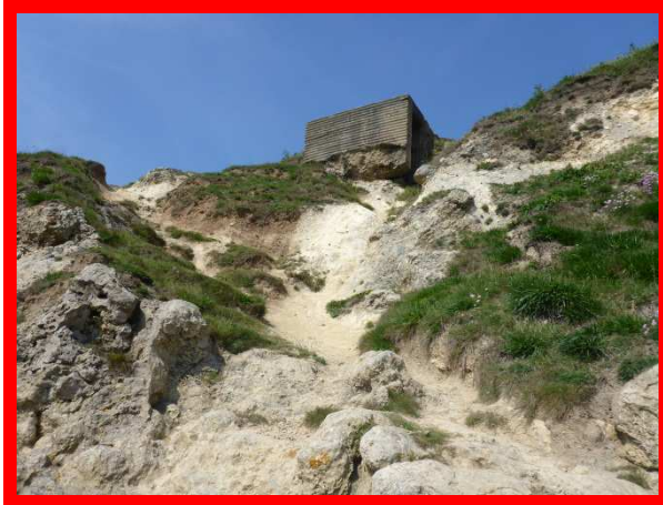
Concrete bunker at northern access ramp to Marsden bay (/0401C04)
