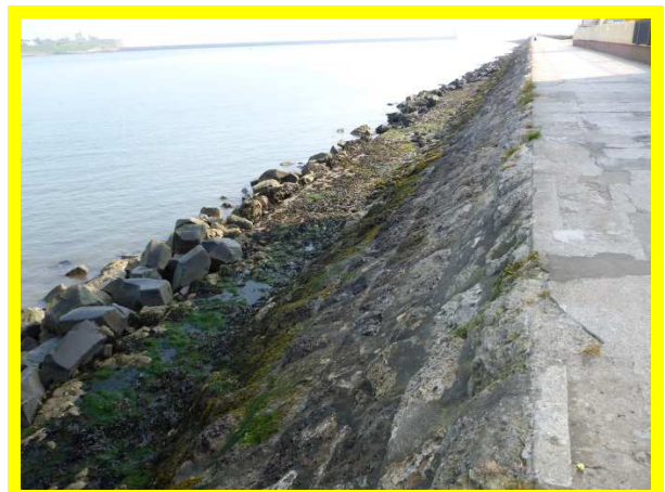
South Pier in overall fair condition along northern face (/0103C01)
