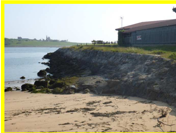
Grouted masonry revetment in fair condition (/0101C01)
