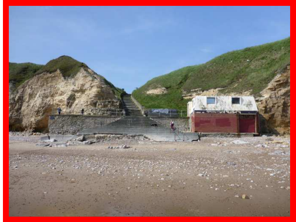
Disused lifeguard station and the Redwell Steps access (/0401C01)
