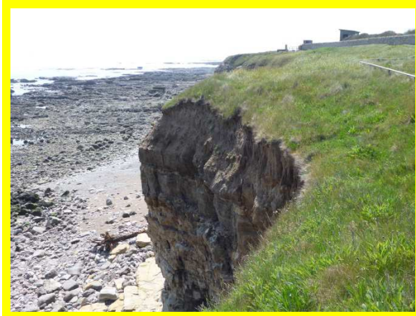
Generally stable cliffs but some local slumps close to footpath at Whitburn nature Reserve (/0502C01)
