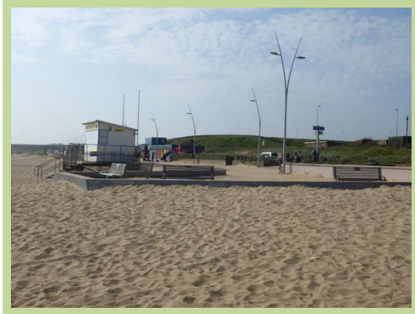
Good condition of reconstructed wall, with high surrounding beach levels (/0201C04)
