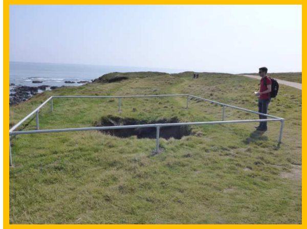
Sink hole south of Man Haven Bay (/0401C04)
