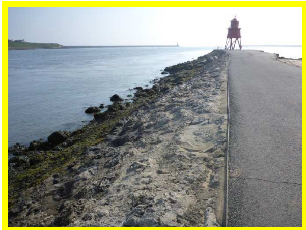
River-facing side of South Groyne in fair overall condition (/0101C02)
